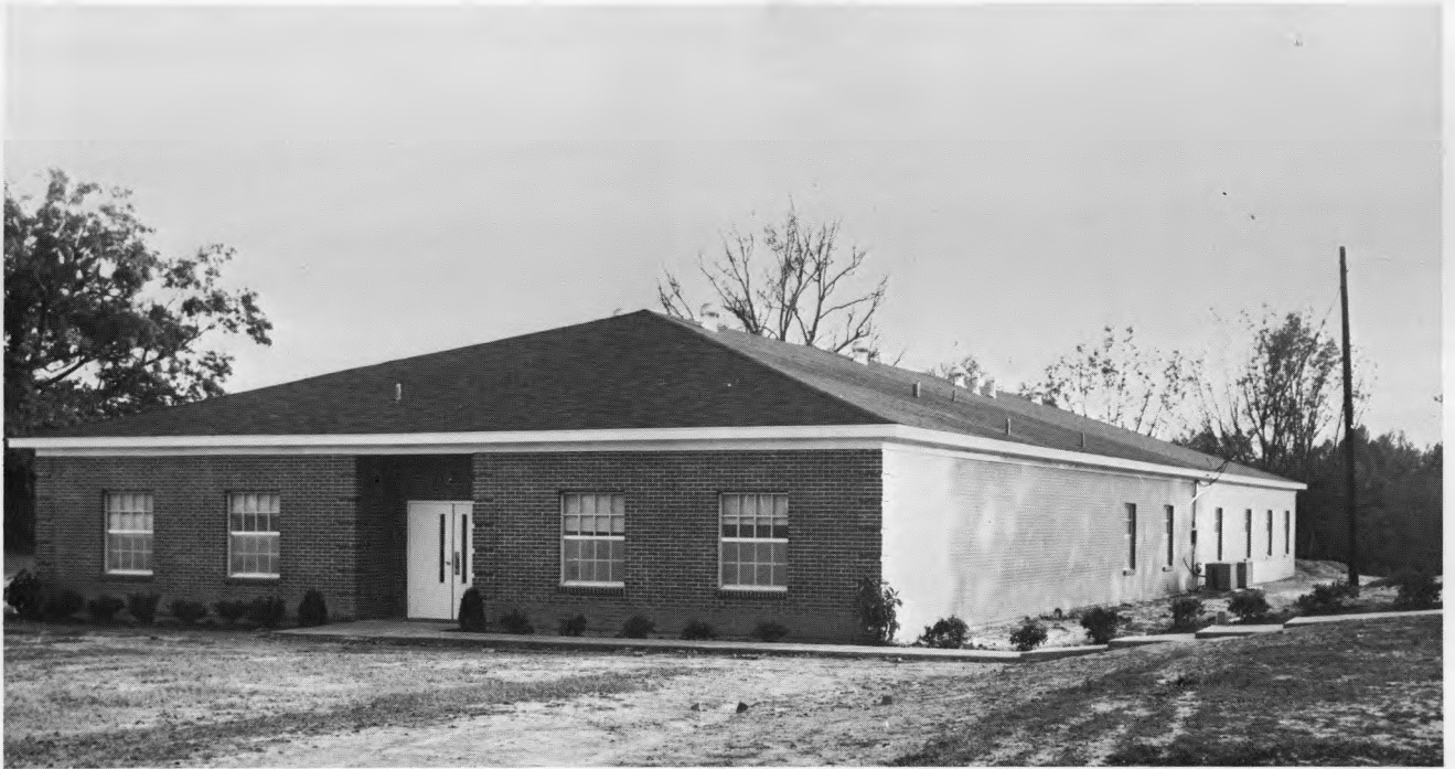
One of the biggest additions to life at CHA this year has been the completion of the Science Building. This facility houses all science and junior high courses.
